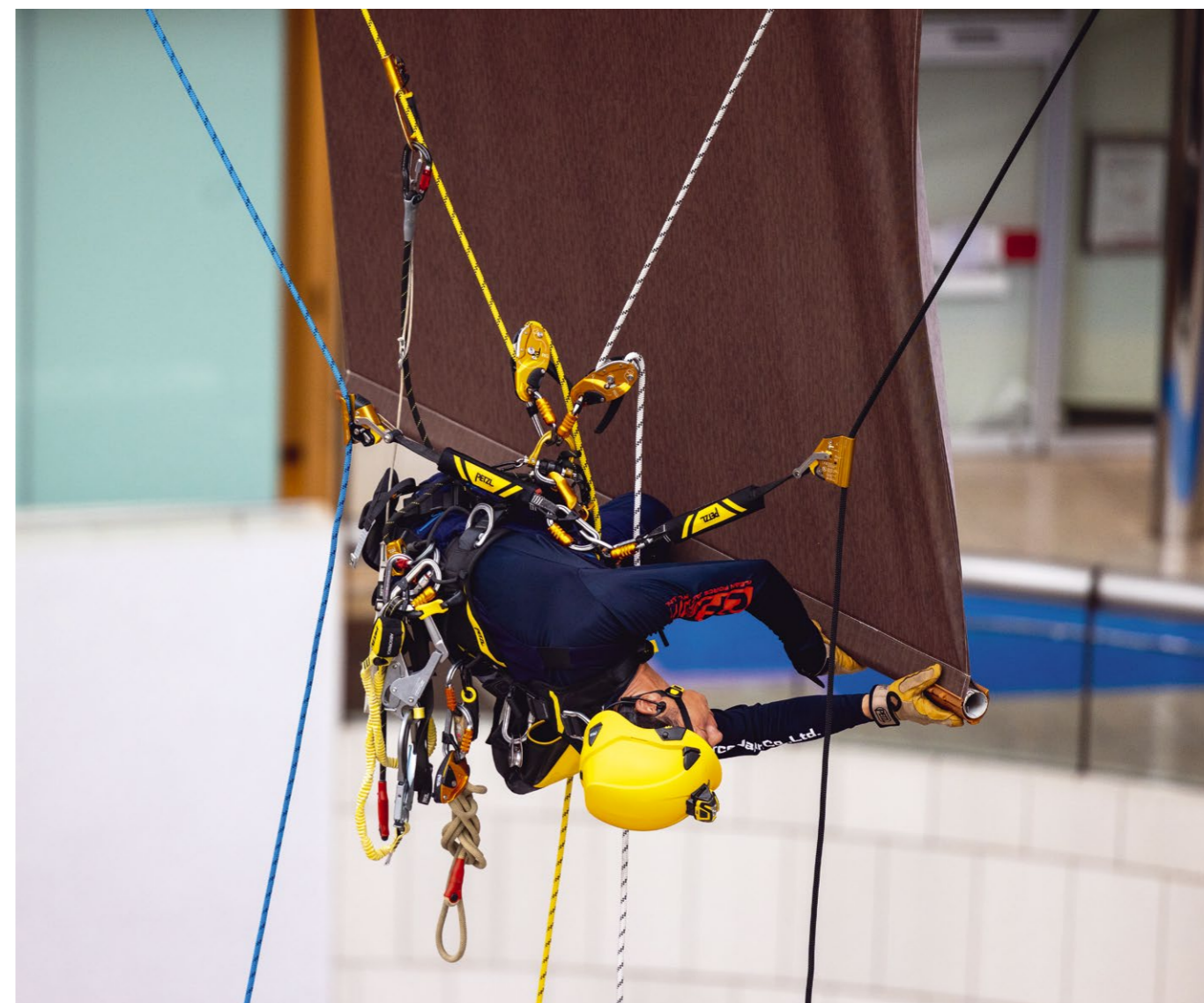
Rope access work at the Tokyo Metropolitan Theater. © 2025 Petzl Distribution - Lafouche - Tokyo Metropolitan Theater - Clean Force Japan
